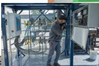
**Mounting the steam distribution control panel**
